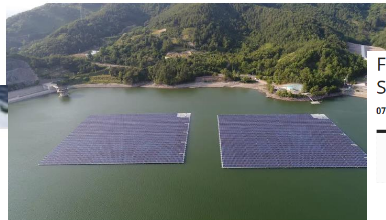
The Geumjeon floating solar power plant, in South Korea. | Seaflex
