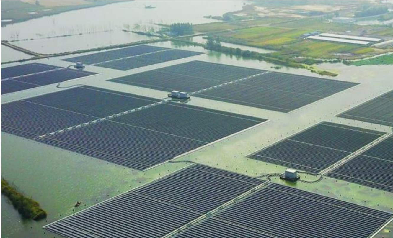
Trina Solar Huaibei Anhui China 40MW Floating Project
