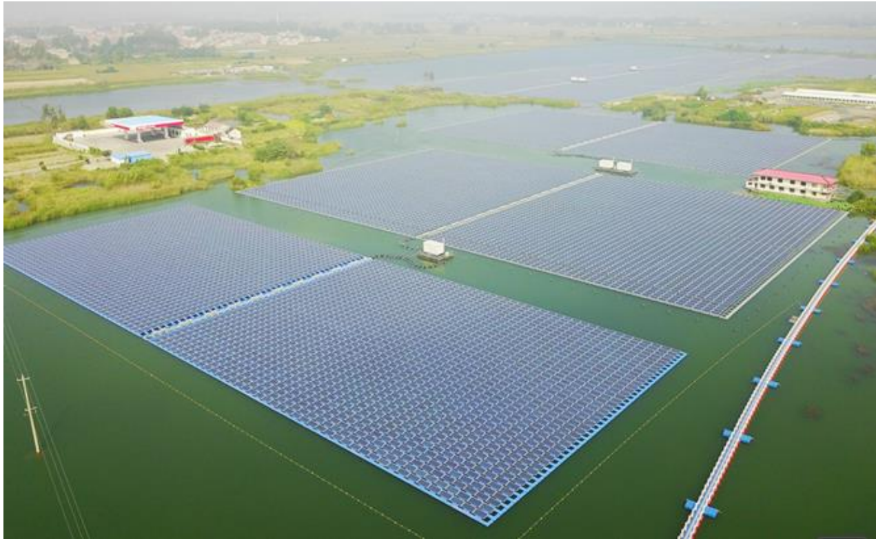
Trina Solar Yingshang 130MW Floating Project World's Largest Floating Project, COD 2019
