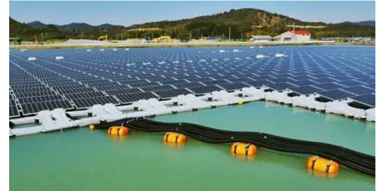
Trina Solar Hyôgo-ken Japan 2.9MW Floating Project
