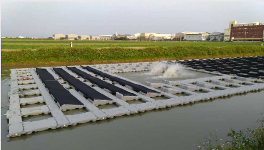
Research for installation of FPV on fish farming and oxigenation
