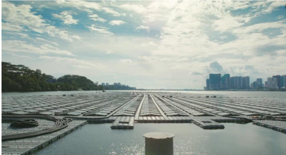
Woodlands Offshore Floating system, 5 MWp
