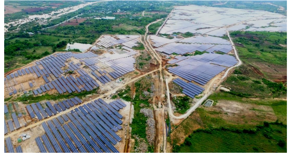
Solar Farm in Vietnam, 168 MWp
