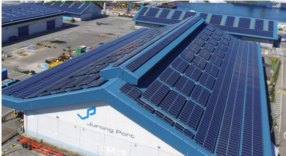
Jurong Port, 9.5 MWp
