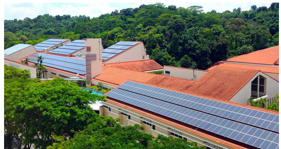
Singapore American School, 1.2 MWp
